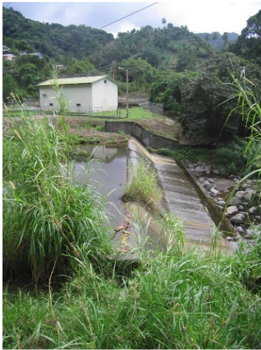
Figure 82. Hydroelectric dam on the Cumberland River at Spring Village.
